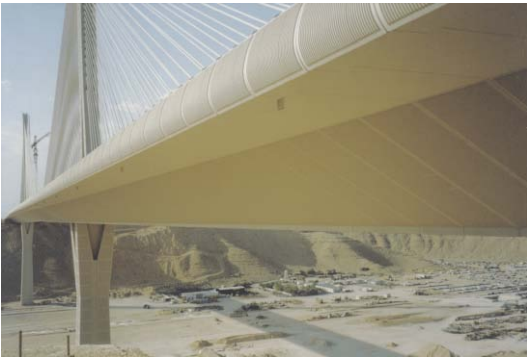
Fig.13.3 Wadi Leban Bridge, Riyadh, Saudi Arabia- General View of The Bridge Looking North
