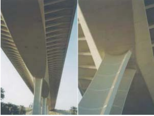
Fig.13.2 Qurashiyah Viaduct, Riyadh, Saudi Arabia- Pier Head and Soffit Finishes Detail
