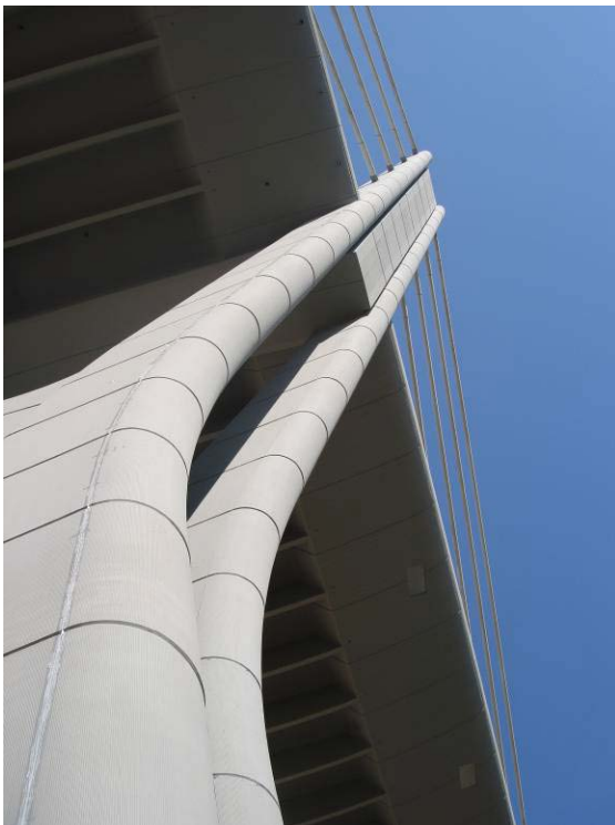
Fig.13.6 Wadi Abdoun Bridge, Amman, Jordan- Development of tower forms & Finished tower
