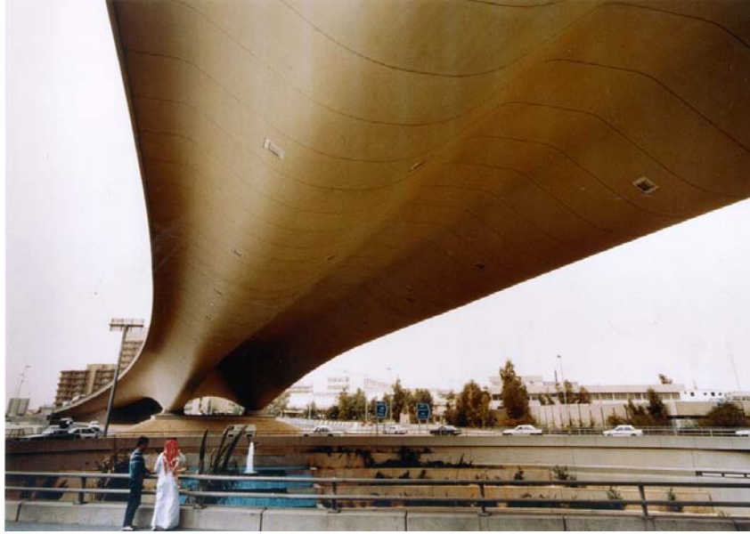
Fig.13.19 Al-Khaleej Viaduct, Riyadh, Saudi Arabia - Three-Tier Interchange Showing Deck Soffit Lighting
