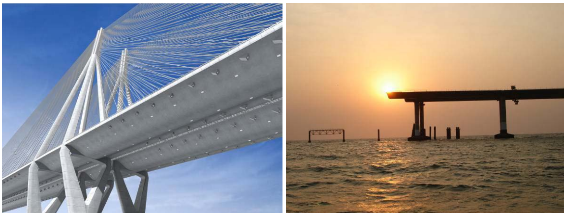
Fig.13.25 Bandra-Worli Sea Link Project, Mumbai, India - Computer Generated Image of The 500m Span Cable Stayed Bridge, and Viaduct Under Construction.
