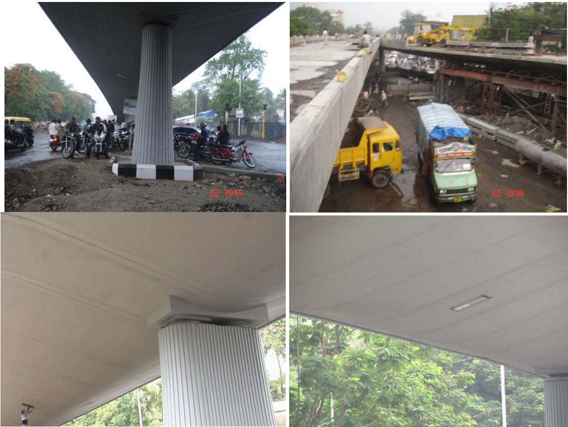
Fig.13.22 University Circle Flyover, Pune.
