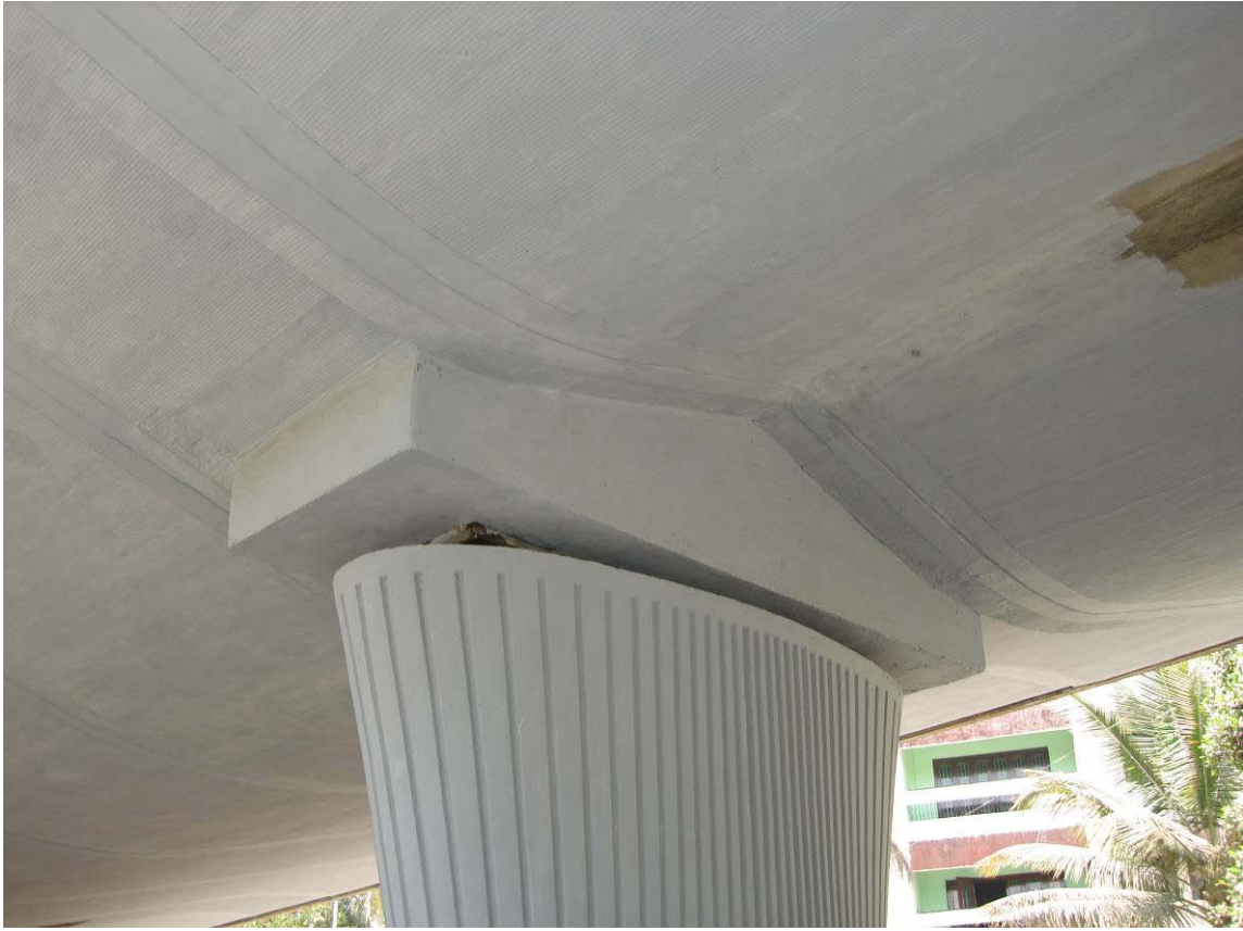
Fig.13.15 Bifurcation Detail, University Circle Flyover, Pune- Top Left: Stitch Detail. Top Right: Construction. Bottom: Root of Bifurcation.
