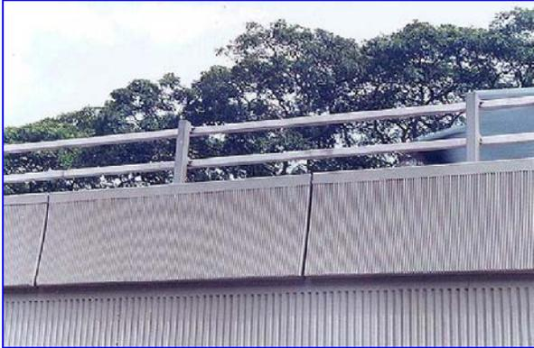
**Fig. 14.14 Example of Precast Architectural Fascia**
