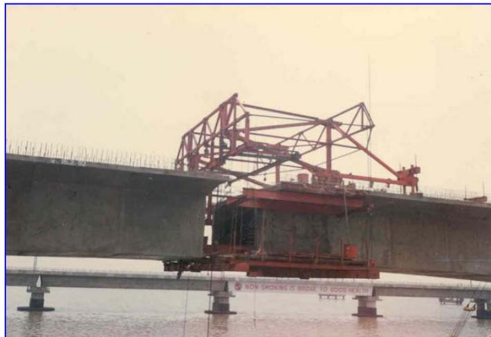
**Fig. 14.22 Cantilever Construction for Second Thane Creek Bridge**
