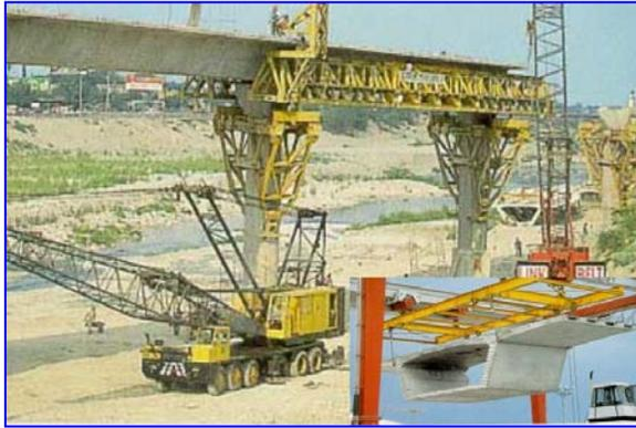
**Fig.14. 5 Precast Segmental Const.**
