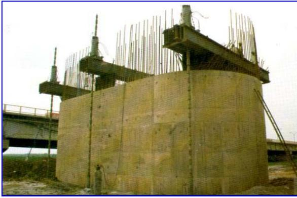
**Fig.14. 12 Jack-down Construction of Well Foundations**
