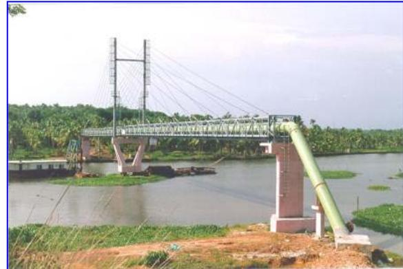
**Fig.14. 13 A Cable-stayed Pipe Bridge at Cochin**
