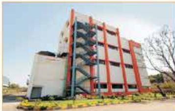
State-of-the-art plant at Ambarnath
