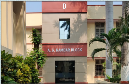
Newly Renovated A. G. Kamdar Block
